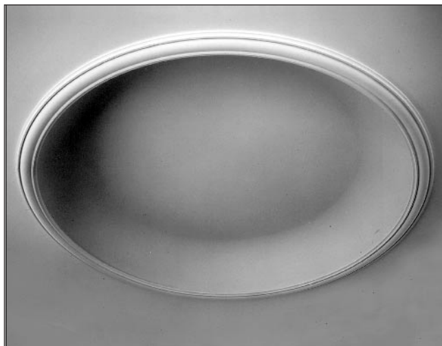
Installed dome with custom dome ring.
