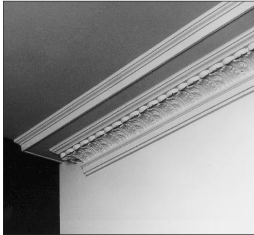
Installation of cornice - 6313
